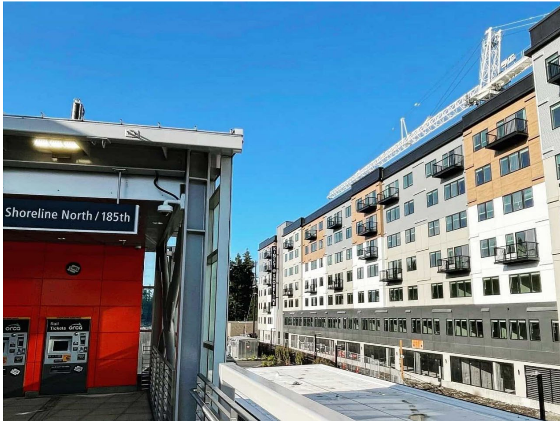
A 298-home, 7-story apartment building next door to a light rail station in Shoreline, Washington, just north of Seattle. Photo by Dan Bertolet, used with permission.
