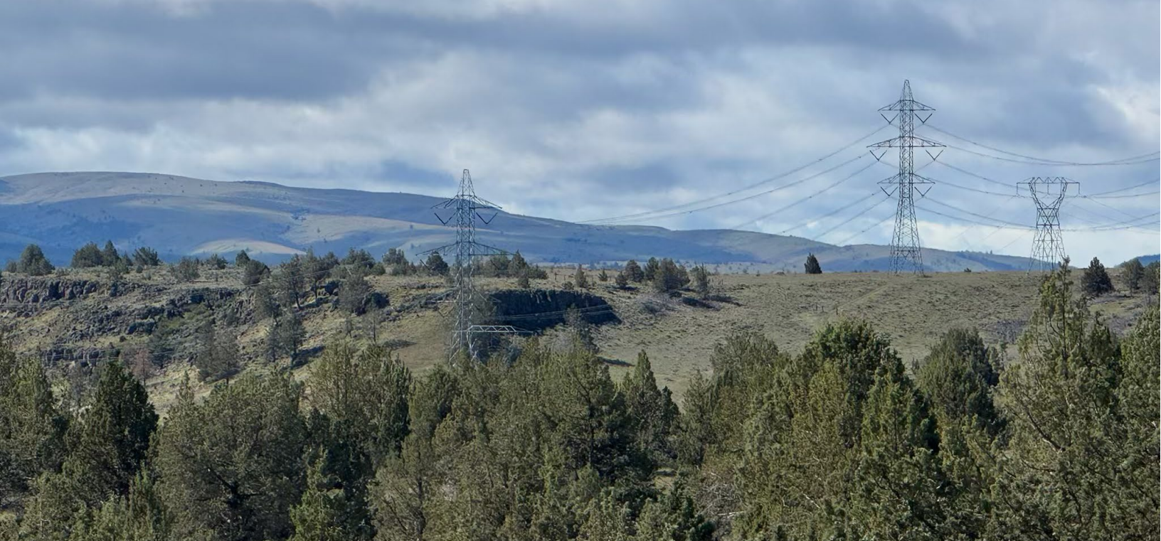
A transmission line runs along the Dalles-California Highway near Maupin, Oregon. Some new transmission lines could run alongside existing corridors.
