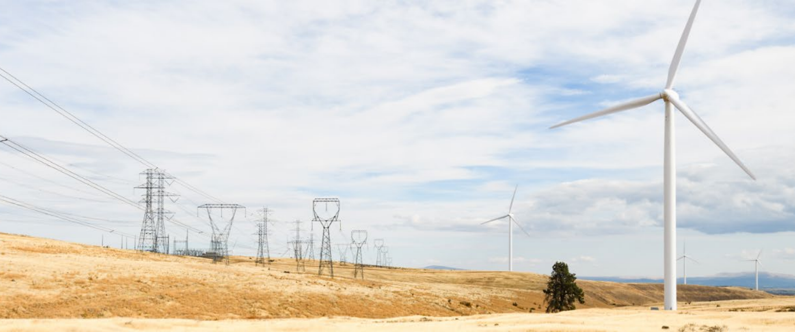
Wind turbines neighbor transmission lines, connecting clean energy to the homes and businesses that need electricity.
