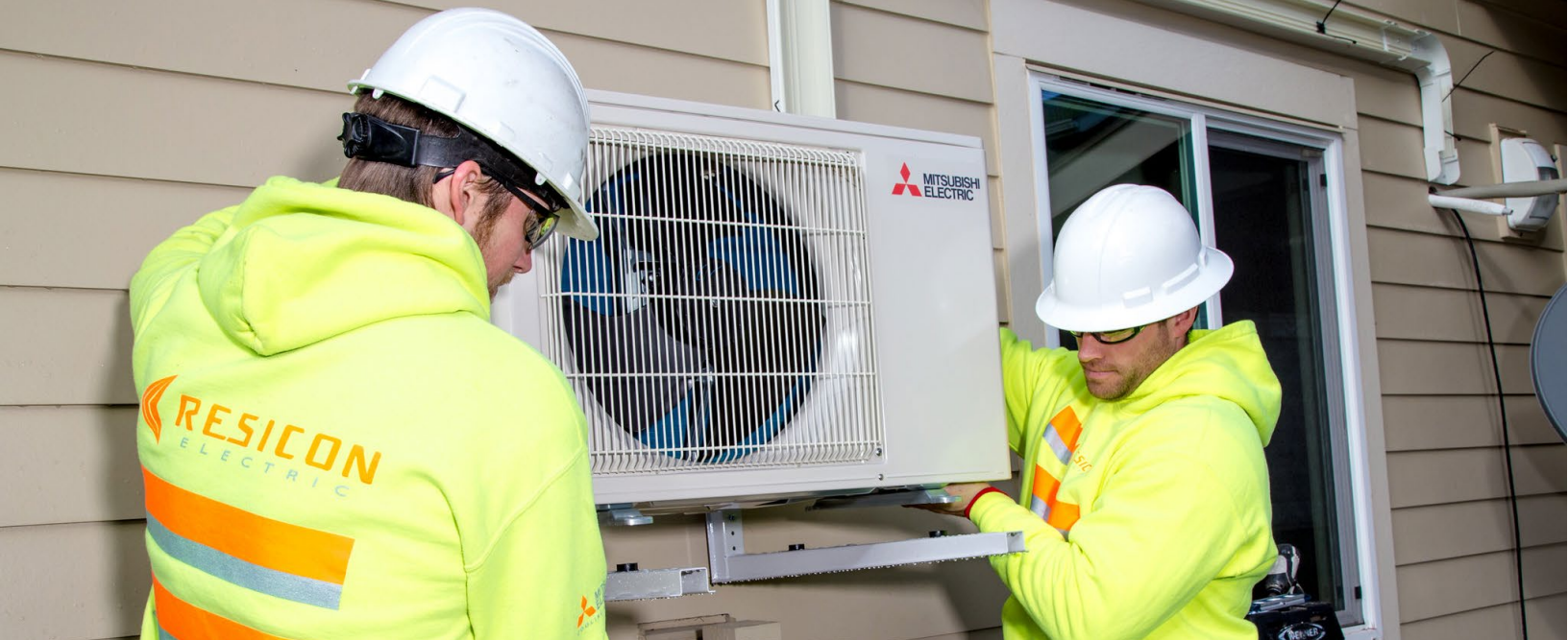
Construction workers help install new heat pumps for residents in south Seattle.
