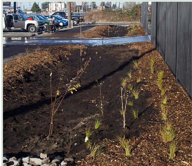
The new swales in front of the Markey Manufacturing Co. catch rainwater runoff that sinks into the ground or is taken up by plants.
