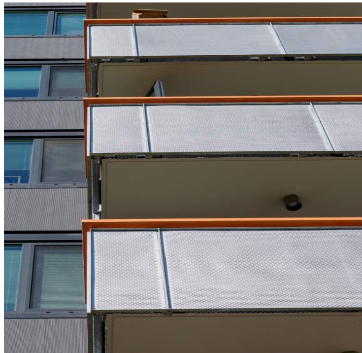
PERFORATED METAL BALCONY GUARDRAILS
